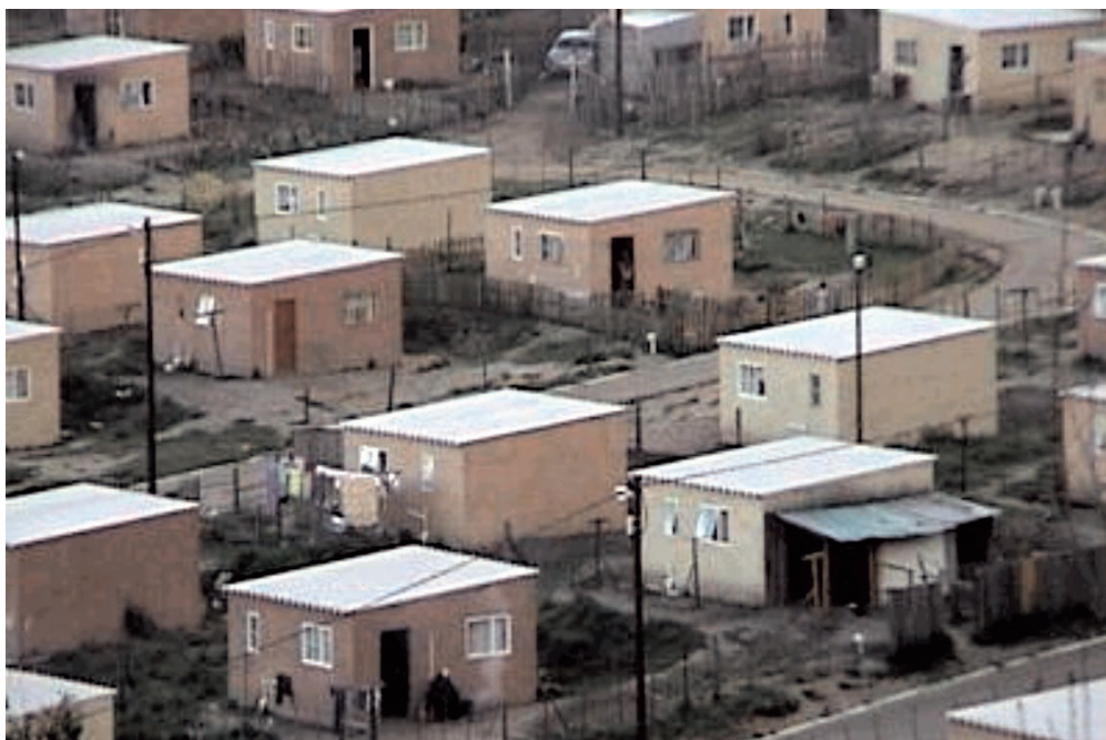
Overview of a typical low income housing estate
