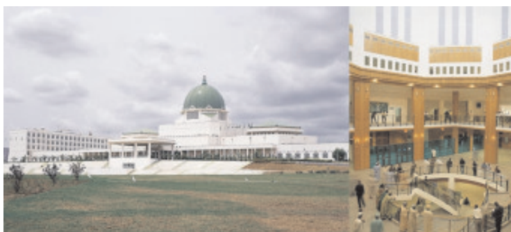
The National Assembly Complex, Abuja
